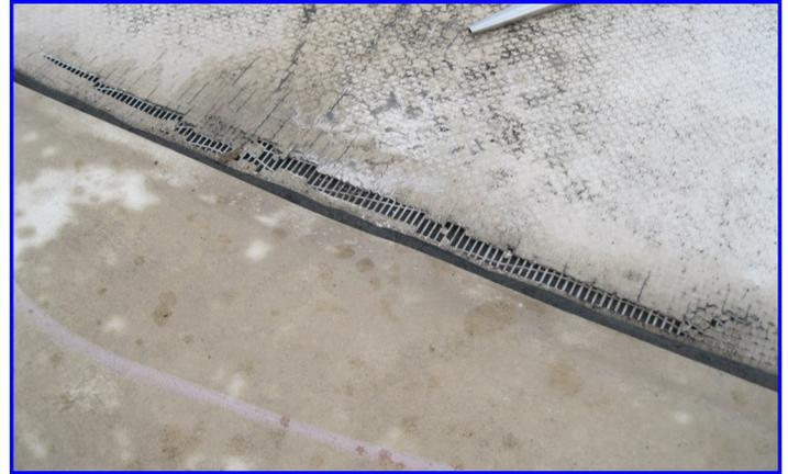
The TPO membrane had worn down to the point that the internal reinforcing fabric was exposed in areas.
